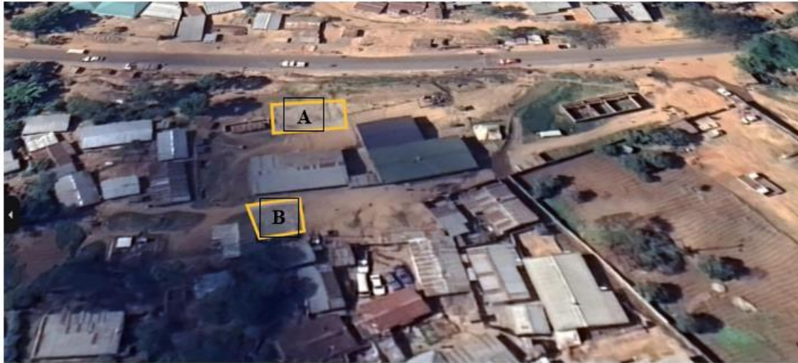
Figure 4: Shows (A) the PSF proposed site and the current ESCOM pole location and (B) proposed new pole location
